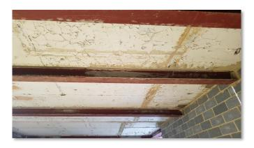
Working in an old Police Station in August 2018, **Grit Blasting UK** completed a re-furbishment project, cleaning by blasting around 100 square metres of supporting steels for the client, a building contractor.
